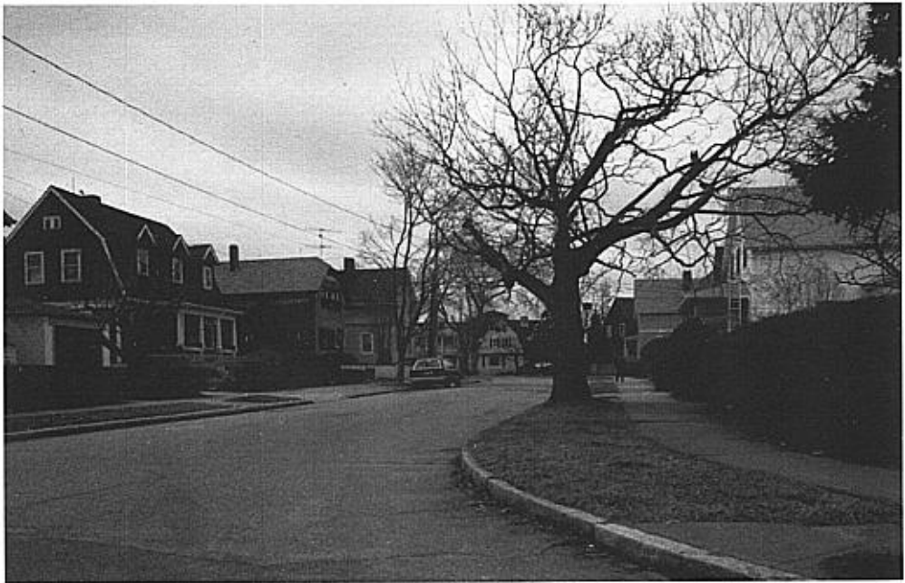
Fig. 2. The Howland Mill Village, 1996. The three workers' cottage designs are all visible at left. The contour plan, the irregular placement of the cottages, the wide streets with granite curbs, and the trees lining the sidewalk are all original design features. Photograph by Kingston Heath.
