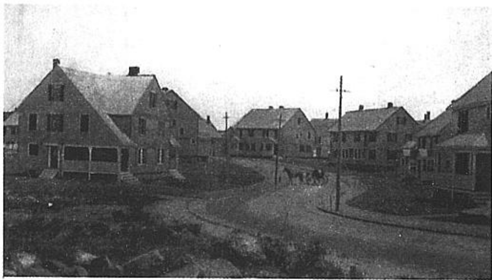
Fig. 17. The housing at Hopedale under construction, about 1898; photograph in Model Factories and Villages (London, 1905).
