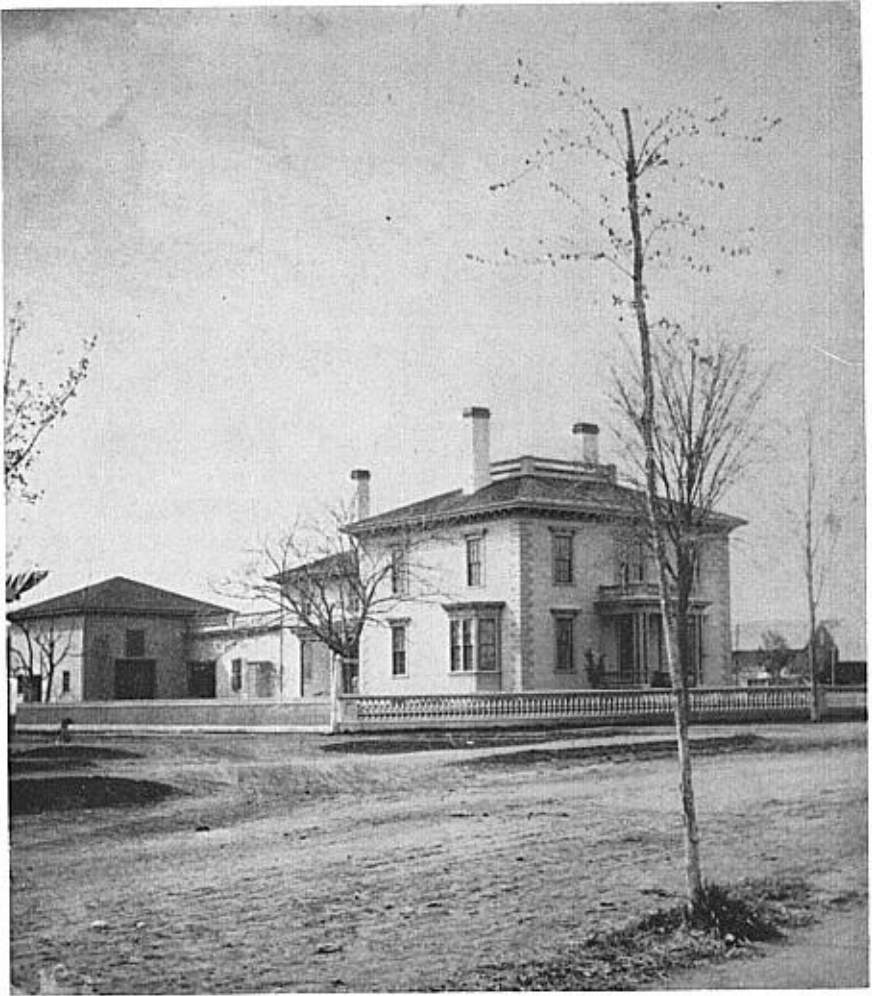
FIG. 11. HOUSE (NOW DEMOLISHED), WATERVILLE, MAINE From a stereograph in the Society's collections, taken probably in the 1870's.
